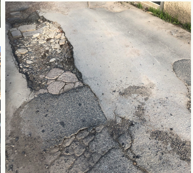
Patched and poor quality hard surfacing
